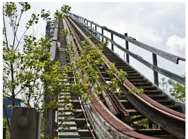
Before demolition of Six Flags almost two decades later (Roller Coaster), KEG-KEG/Shutterstock (2024)
